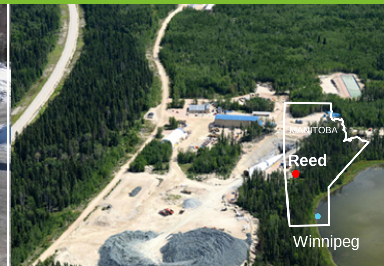
Aerial view of Reed project site
