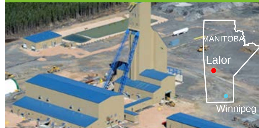
Aerial view of Lalor project site
